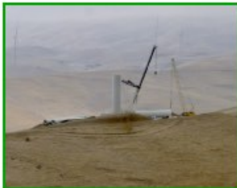
Wind mills basking in the sun. Wind mills under construction.
